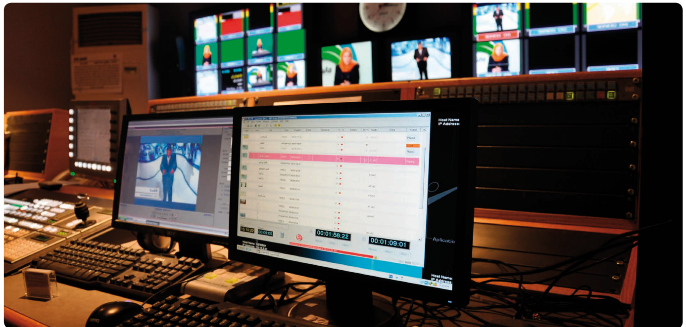
Al Kout TV Studio Control Room
